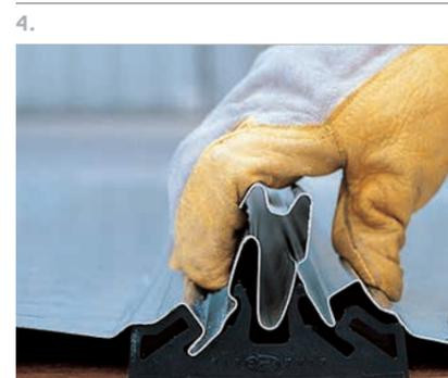
4. Place the overlapping edge of the next panel into the clip by repeating step 1.
