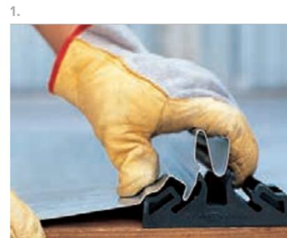
1. Once the panel is completely secured to the first run of clips, insert the second run of clips to the free side of the panel (gutter side for Riverclack® 500 and Riverclack® 550, overlapped side for Riverclack® Grip 600).
