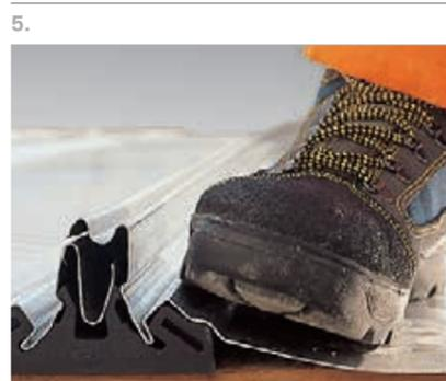
5. Stand on top of the profile to ensure the panels are properly connected.
