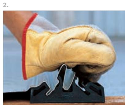
2. Push down carefully on the top until the panel locks into the clip (you should feel a "click"). The panels themselves determine the correct location of the clips.
