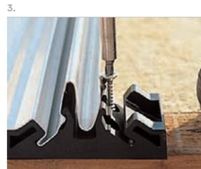
3. Secure the clips to the supporting element using the appropriate fixings.
